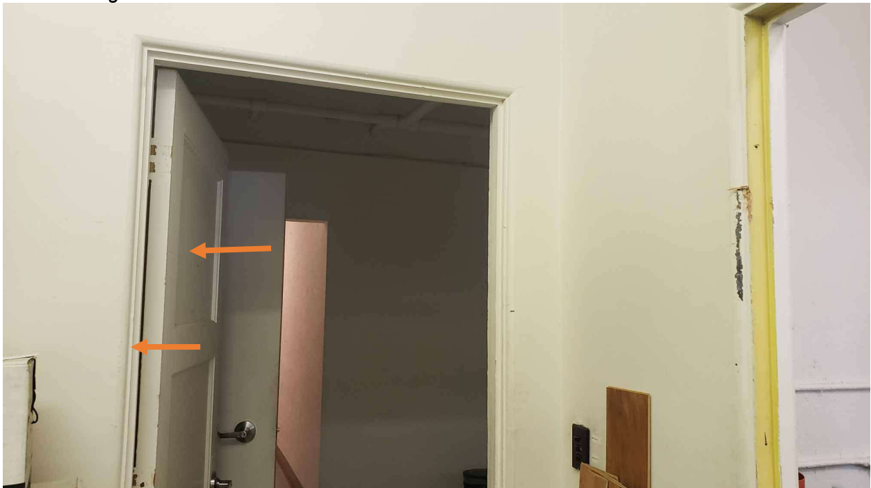
Photo 4: Door frame to hallway in Classroom 2 (sample PB-32,) contains LBP at a concentration of 1.8 mg/cm 2 . The door from Classroom 2 to the hallway also contains LBP at a concentration of 1.4 mg/cm 2 .
