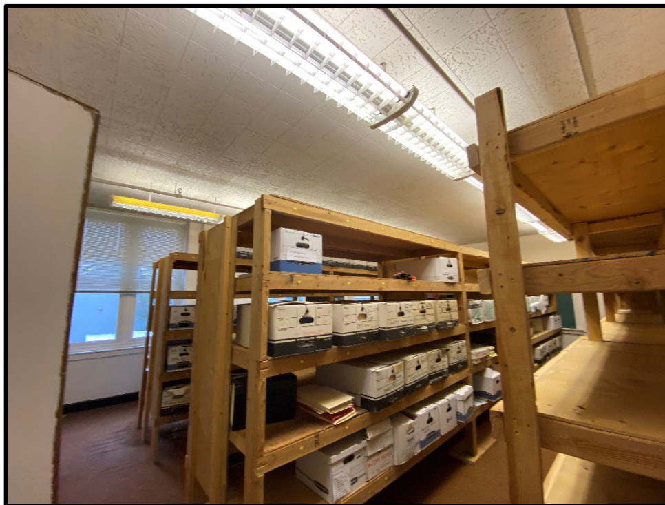
Photo 2: Classroom 2 has one layer of carpet over ACM flooring tiles
