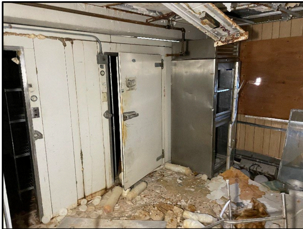
Photo 12: From left to right: walk-in refrigerator (R-13), walk-in freezer (R-14), standup refrigerator (R-15) – Penthouse floor
