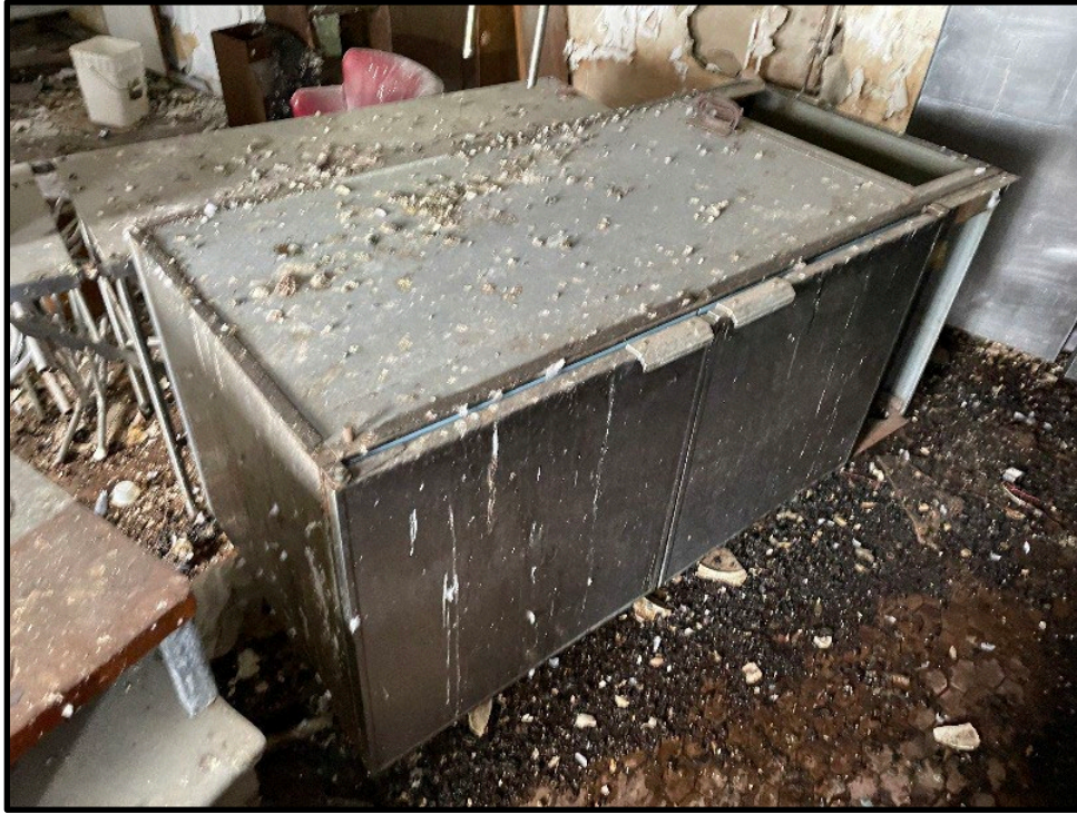
Photo 21: Chest freezer (R-22) – Penthouse floor
