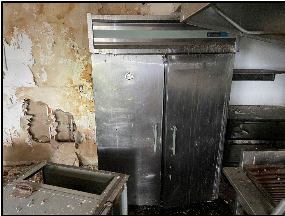
Photo 22: Standup refrigerator (R-23) – Penthouse floor
