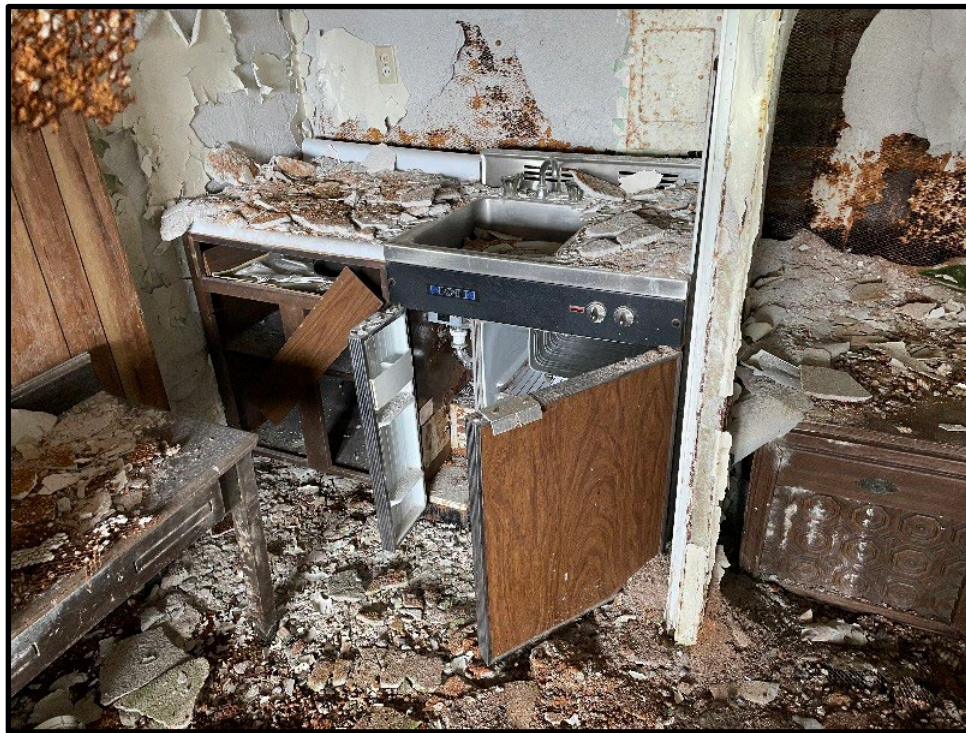
Photo 10: Mini-fridge / Kitchen unit (R-12) – 10 th floor
