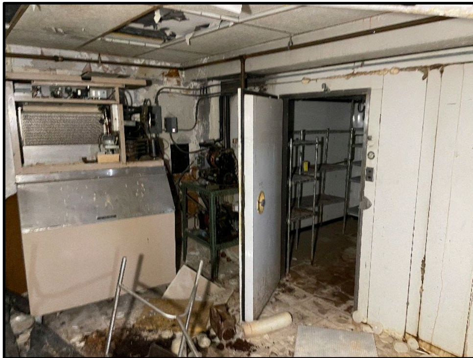
Photo 14: From left to right: Ice machine (R-16), walk-in refrigerator (R-13) – Penthouse floor
