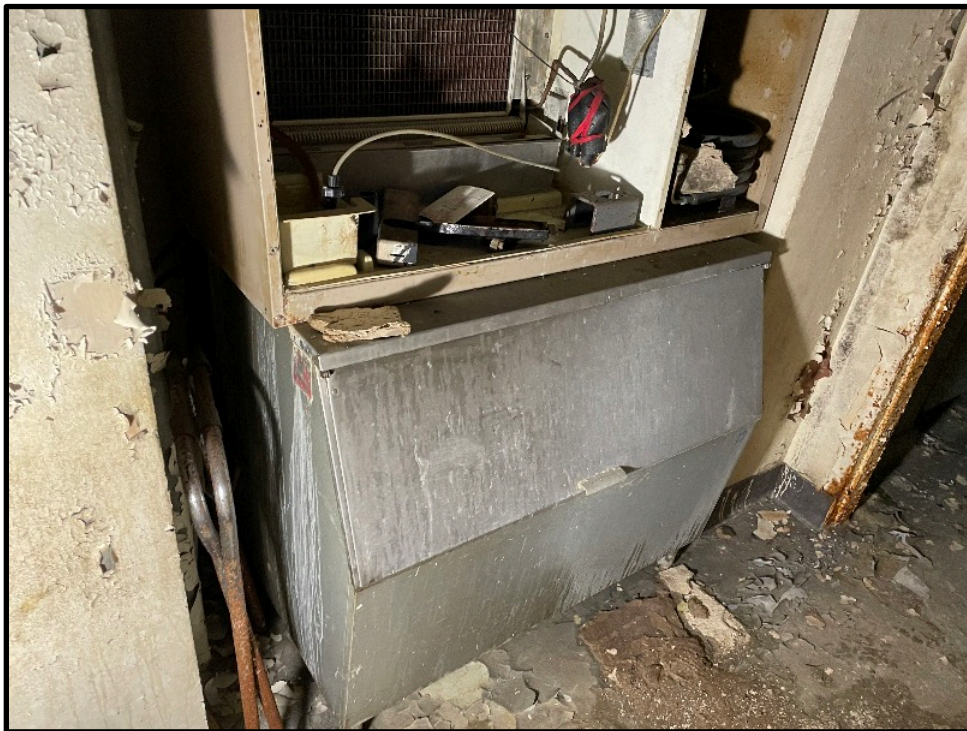
Photo 8: Ice machine (R-6) – Ground floor
