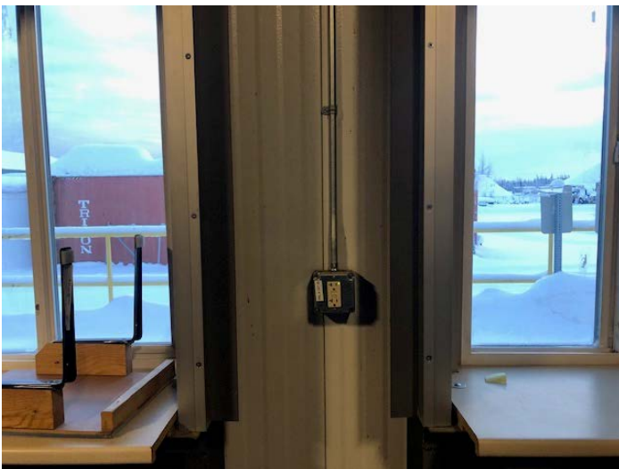
Existing power outlets
