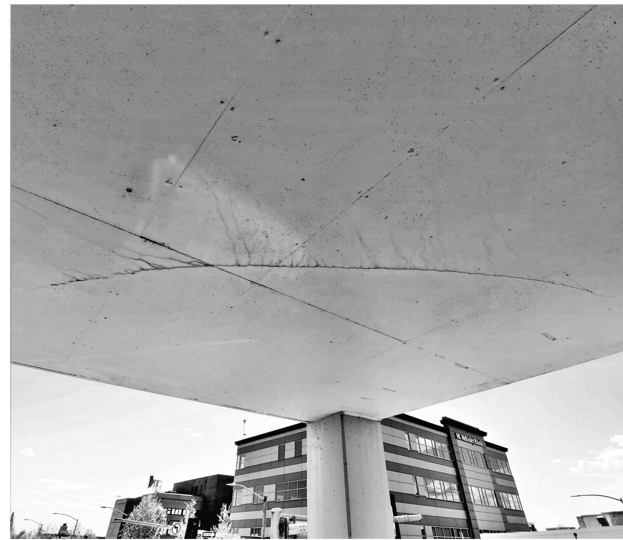
3.A REPAIR 3 - POST TENSIONED SLAB CRACKING S201 1" = 1'-0"
