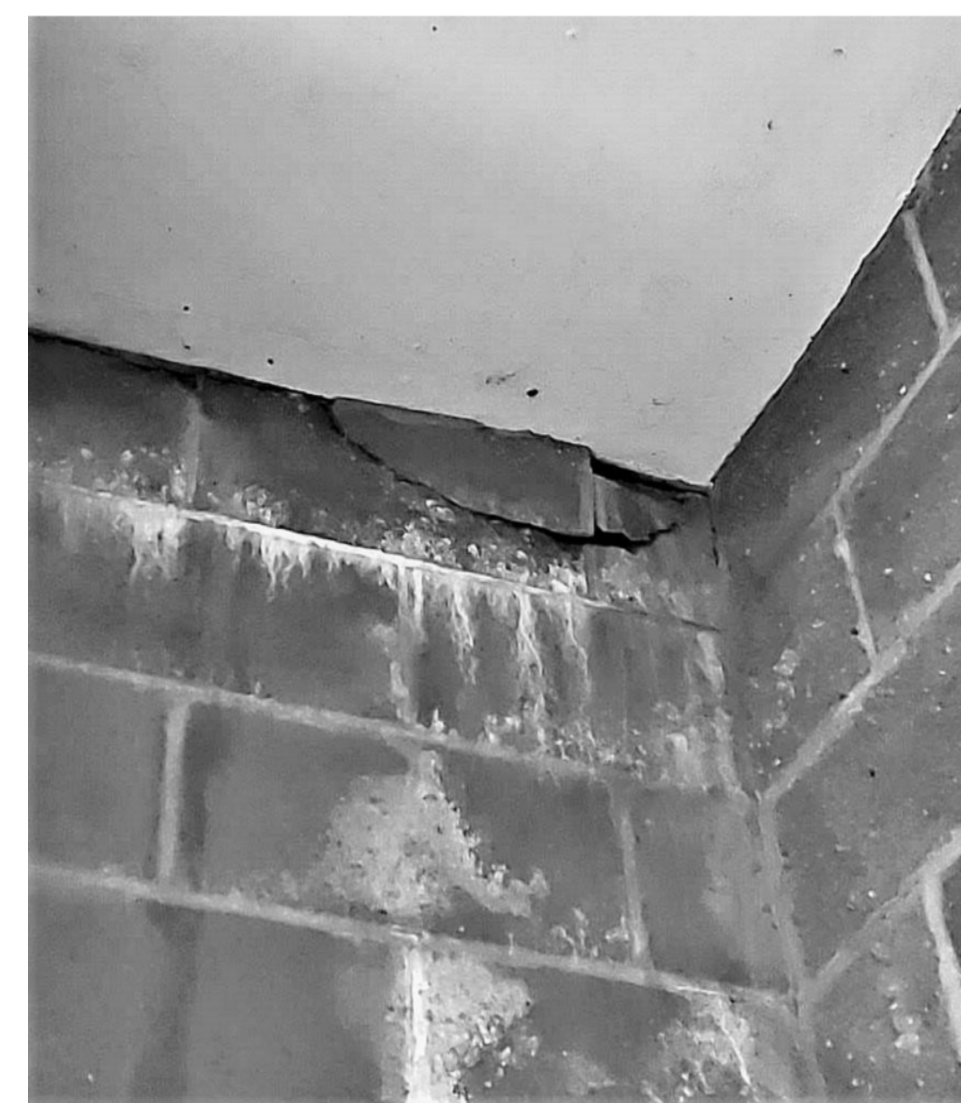
6 REPAIR 6 - CRACKED CMU FACE SHELL S201 1" = 1'-0"
