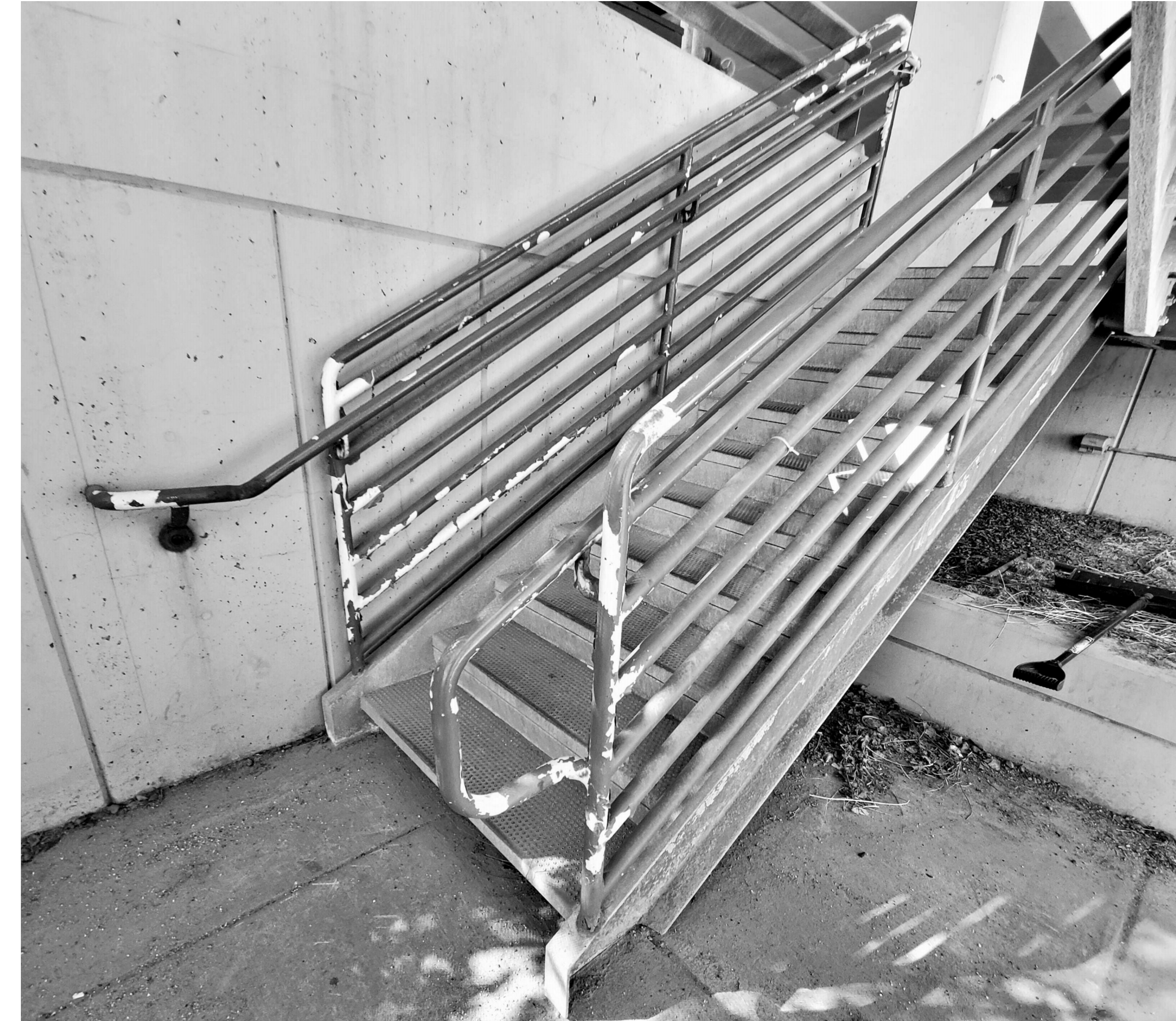
A1.B S202 ALTERNATE #1 - REPAIR A1 - STAIR CORROSION 1" = 1'-0"
