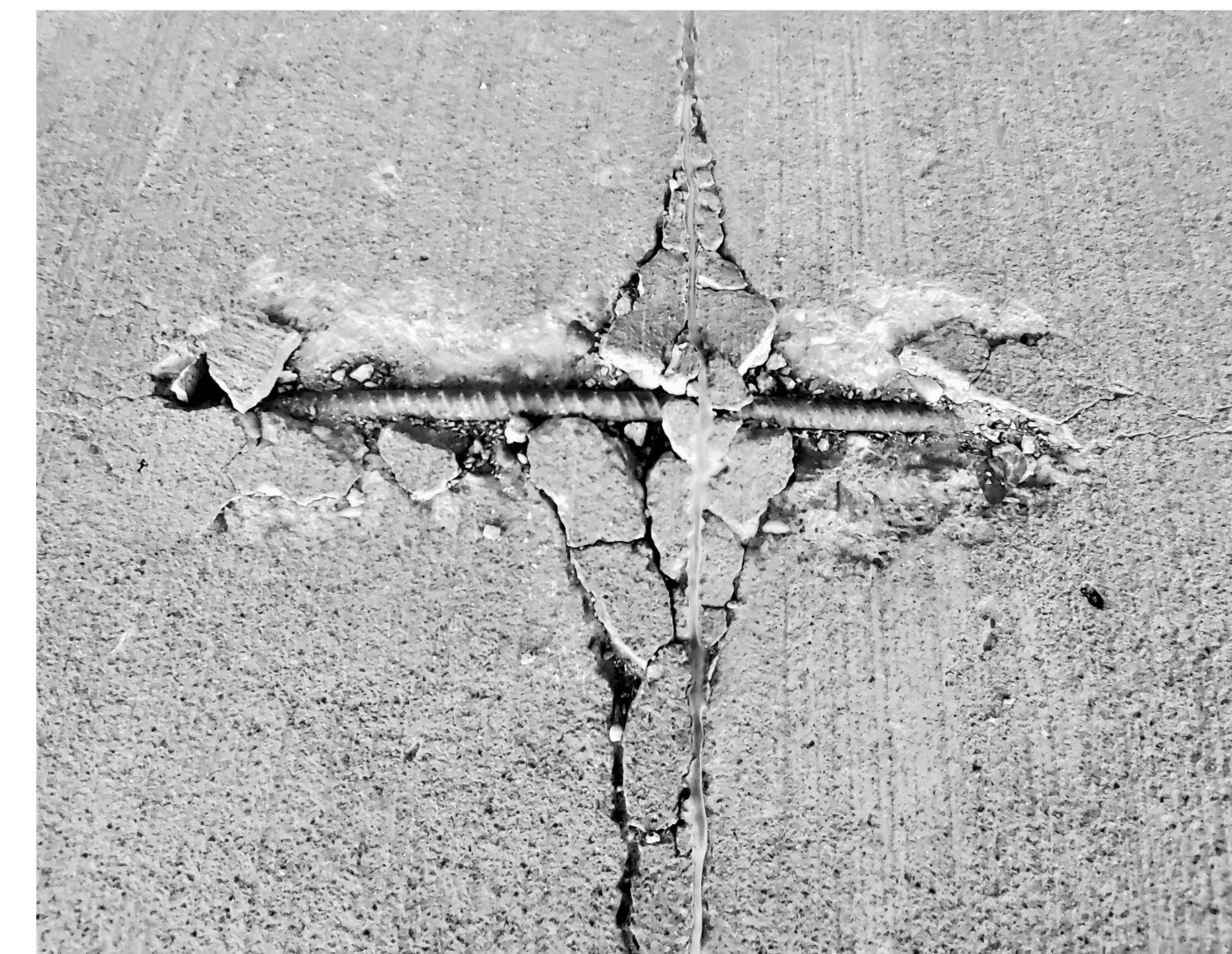
8 REPAIR 8 - DIAMOND SPALLING OF SLAB S201 1" = 1'-0"
