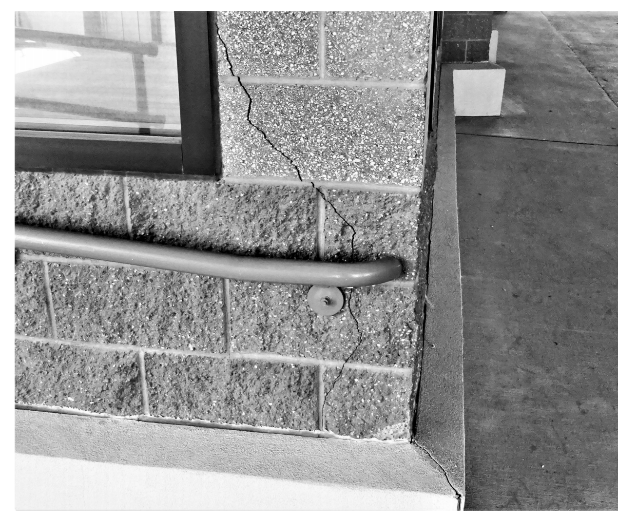
4.A REPAIR 4 - CMU CRACKING (FACE) S201 1" = 1'-0"
