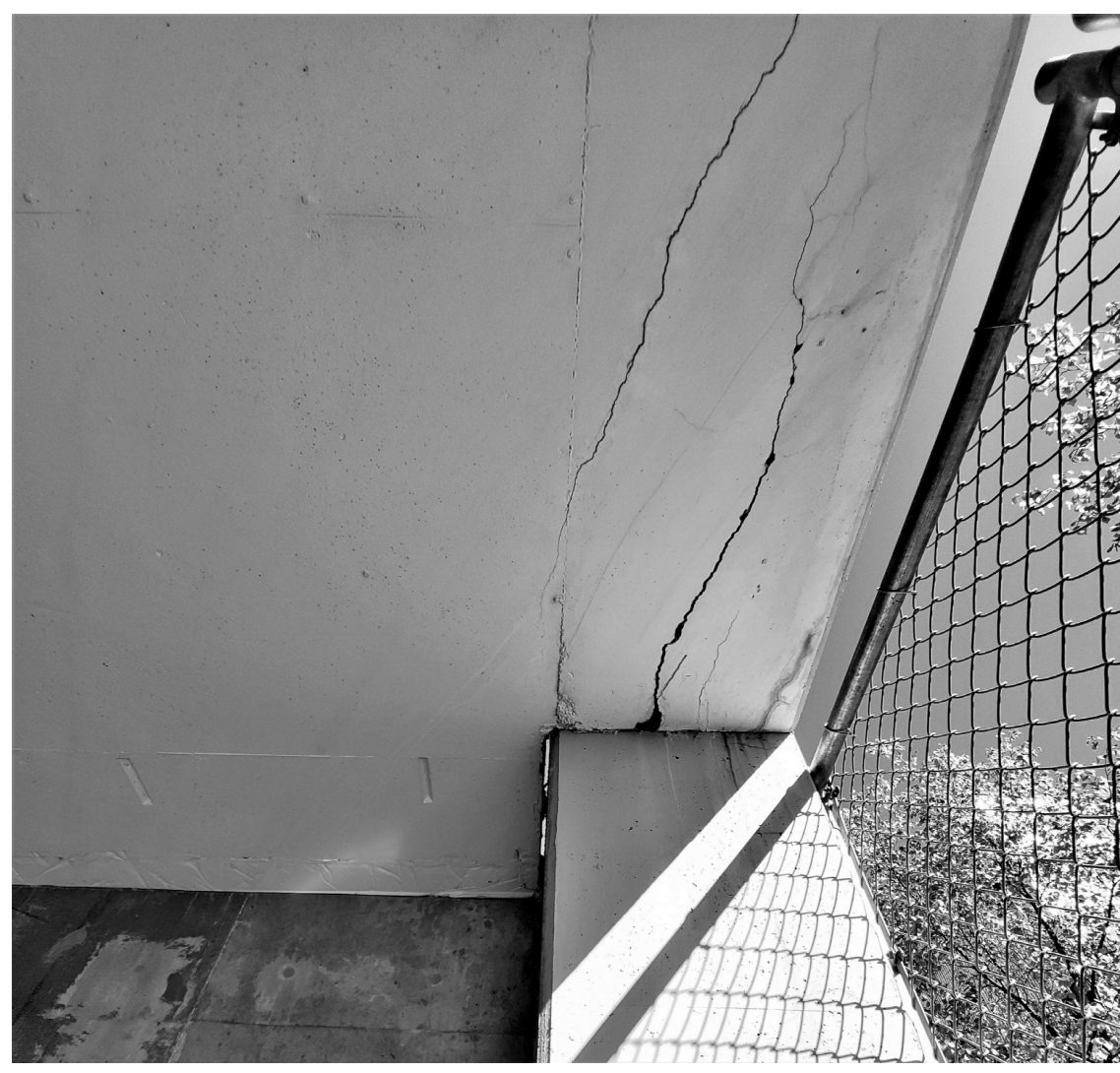
1.B REPAIR 1 - SPANDREL BEAM CRACKING (BELOW) S201 1" = 1'-0"
