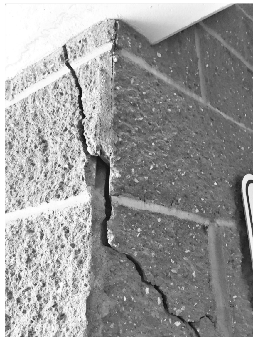
5 REPAIR 5 - CMU CRACKING (CORNER) S201 1" = 1'-0"
