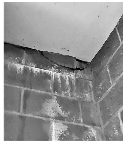
6 REPAIR 6 - CRACKED CMU FACE SHELL S201 1" = 1'-0"
