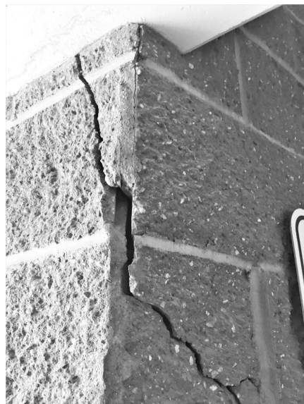
5 REPAIR 5 - CMU CRACKING (CORNER) S201 1" = 1'-0"
