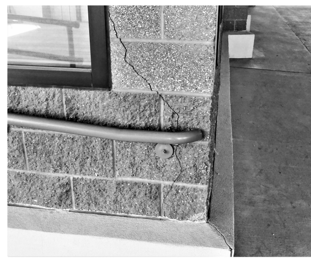
4.A REPAIR 4 - CMU CRACKING (FACE) S201 1" = 1'-0"
