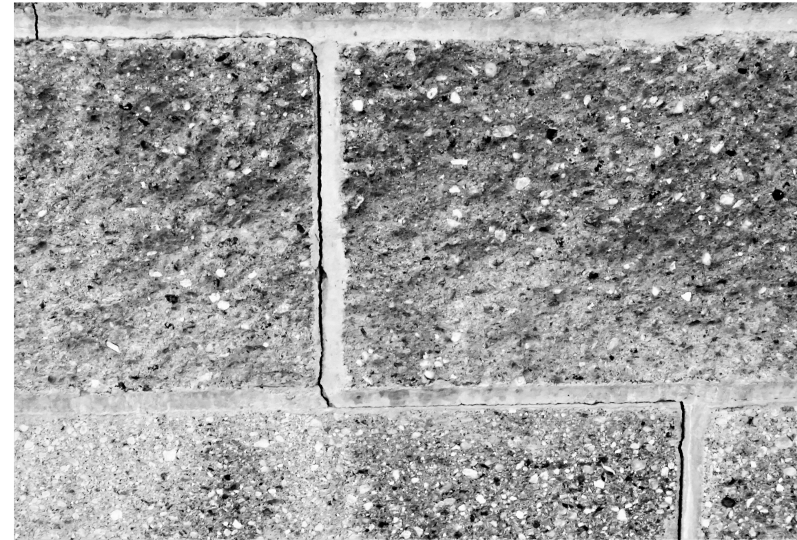
A2 S202 ALTERNATE #2 - REPAIR A2 - CRACKED MORTAR JOINTS AT EXTERIOR CMU FACE 1" = 1'-0"
