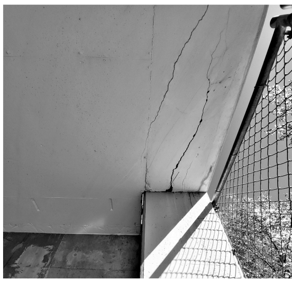
1.B REPAIR 1 - SPANDREL BEAM CRACKING (BELOW) S201 1" = 1'-0"
