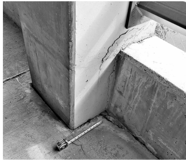
1.A REPAIR 1 - SPANDREL BEAM CRACKING (ABOVE) S201 1" = 1'-0"
