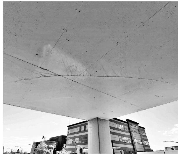
3.A REPAIR 3 - POST TENSIONED SLAB CRACKING S201 1" = 1'-0"
