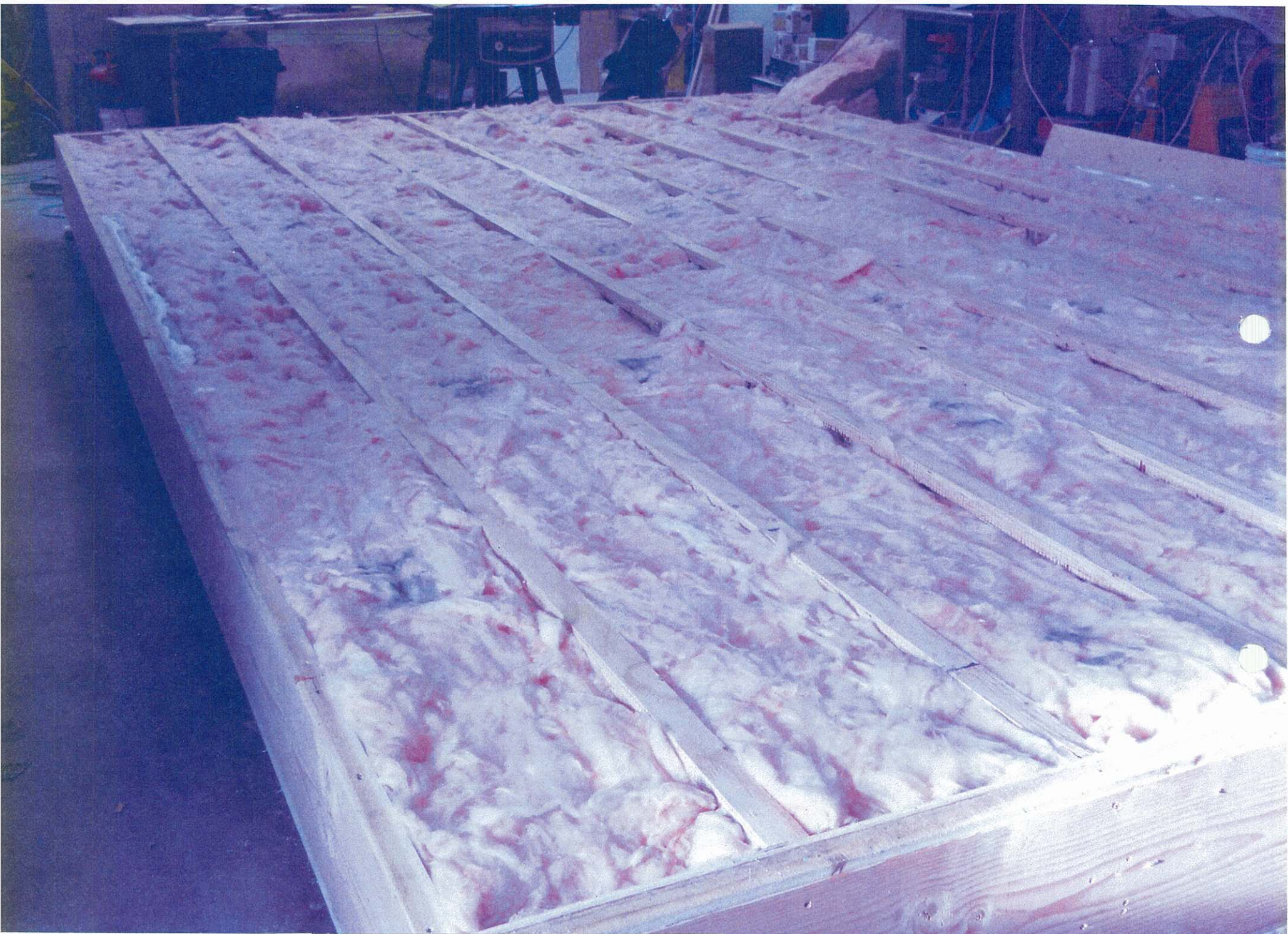
typical view of floorAccessory bldg R-38 insulation 341 Antoinette AGENDA PACKET - February 27, 2012
