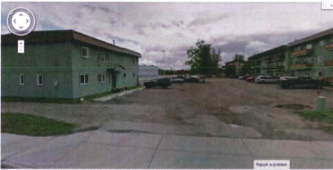
2013 Google Maps: Parking appears to be paved, but in bad shape.
