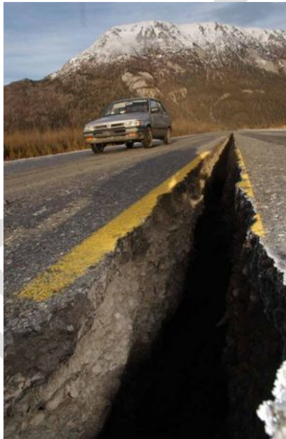
Figure 8-1: Denali Earthquake Road Damage
