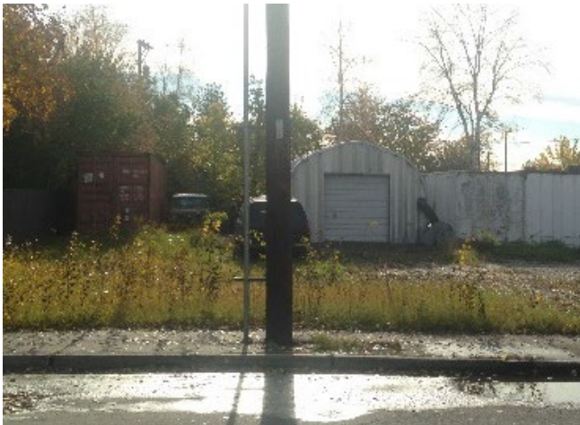
Figure 30. Utility poles placed in the middle of sidewalks make it difficult to walk safely.
