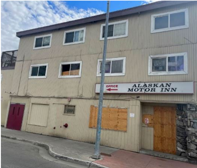
Figure 15. Many vacant buildings need repairs or upgrades.
