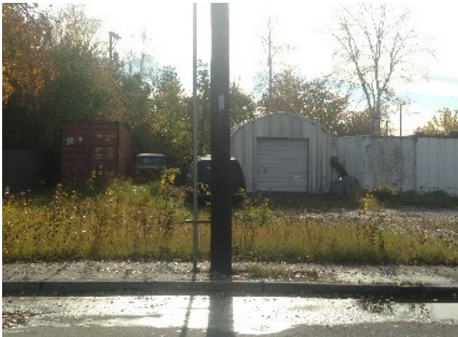
Figure 32. Utility poles placed in the middle of sidewalks make it difficult to walk safely.
